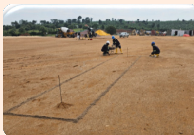
Marking for in-situ duct banks in progress
