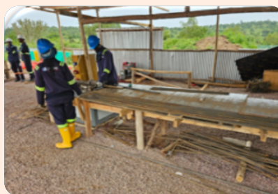
Cut and bend rebars for EITS building in progress
