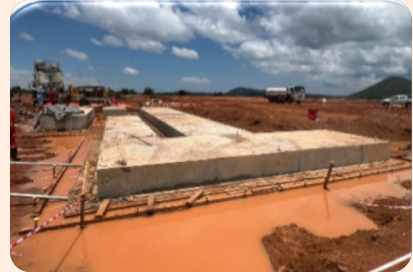
Inlet Custody metering package foundation
