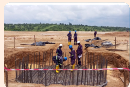
Rebars installation for utility water storage tank in progress
