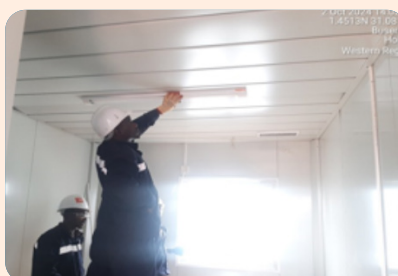
Fixing Fluorescent fitting for single bedroom
