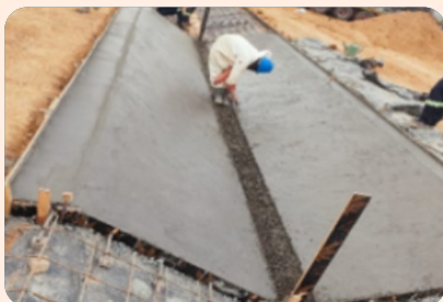
Perimeter ditch drainage
