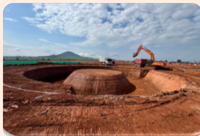
Fire water tank foundation
