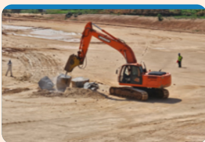
Rock breaking activity in progress
