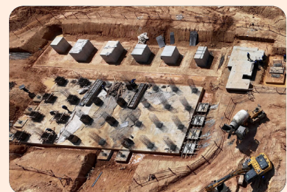
Formworks fixing for pipe bridge foundation in progress
