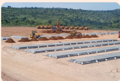
PIPE YARD - Pipe berm construction
