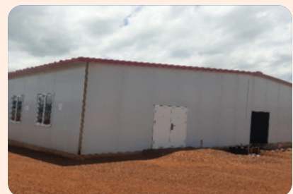
Canteen / mess hall building
