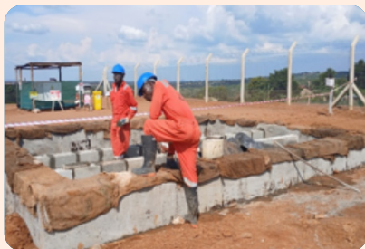
Electrical room foundation
