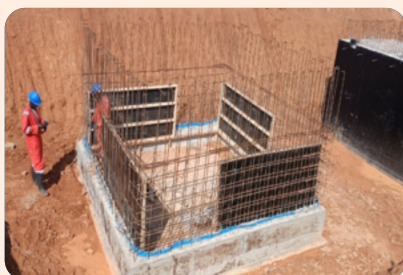
Fixing formwork at the shaft tank
