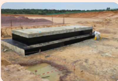
Bitumen coating application for export A, B & C in progress
