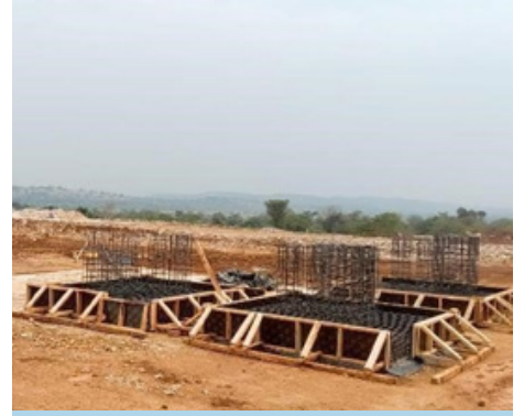
PS-3 Pig Launcher & Receiver rebar fixing
