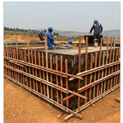
MCPY-6 Holding Tank rebar fixing
