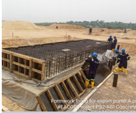
PS-2 Export Pump A formwork fixing
