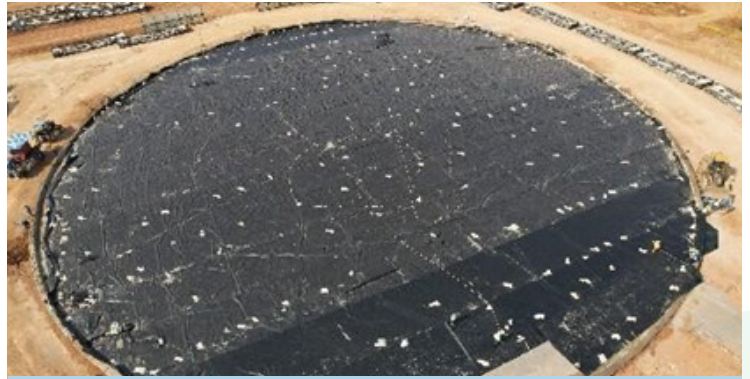
Tank D HDPE installation
