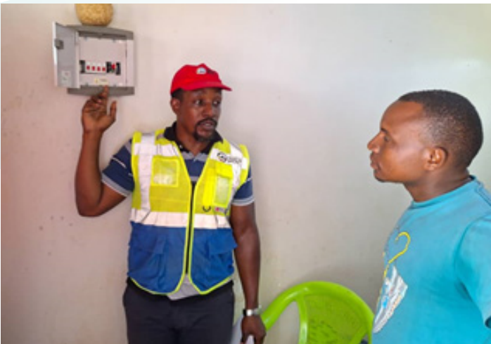
Explaining to the PAP on the function of the circuit breaker.
