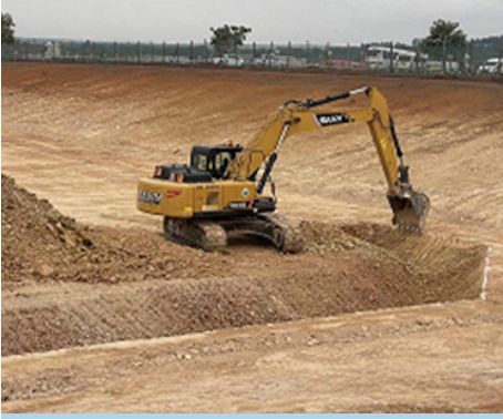
PS-1 Perimeter Ditch construction
