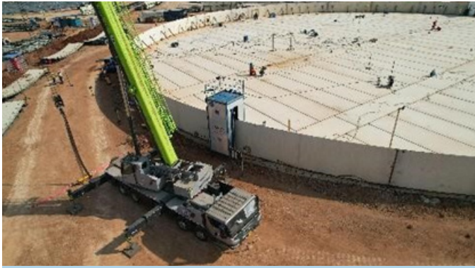
Tank A vertical seam welding
