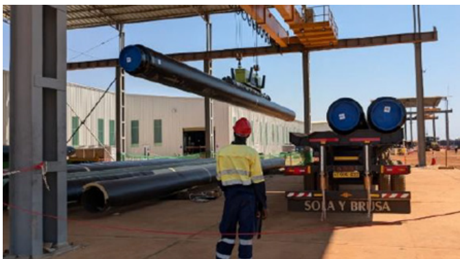
TIS pipe loading
