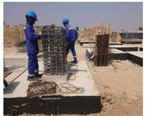
PS-6 Pipe Support foundations
