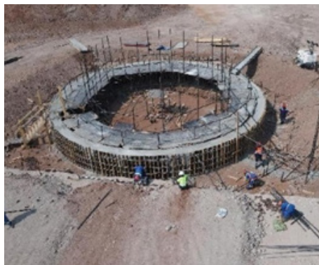
PS-5 Diesel fuel tank foundation scaffold removal
