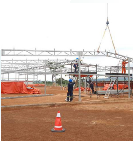
MC-PS1 CTR Canteen roof trusses installation
