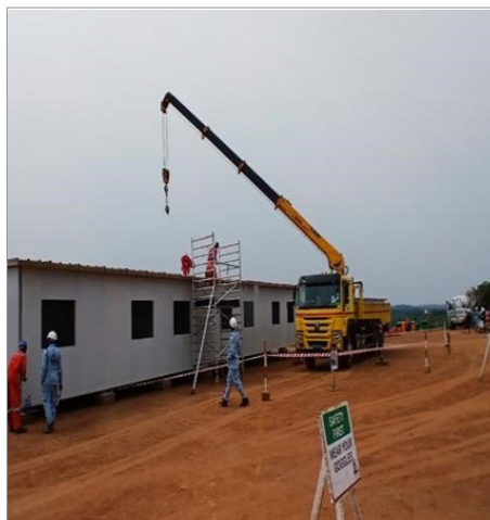
MCPY-3 Portacabin roof fixing
