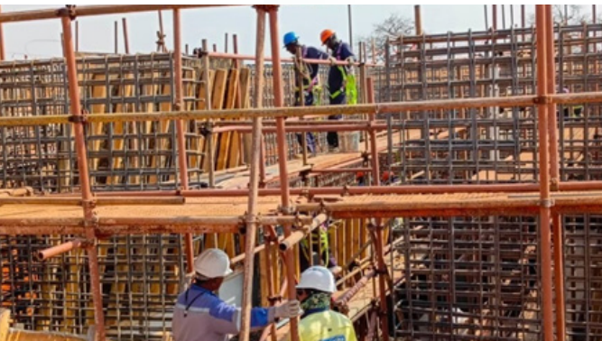
PRS-1 CDD formwork
