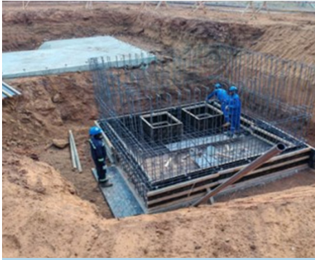
MCPY-7 Shaft Tank rebar fixing
