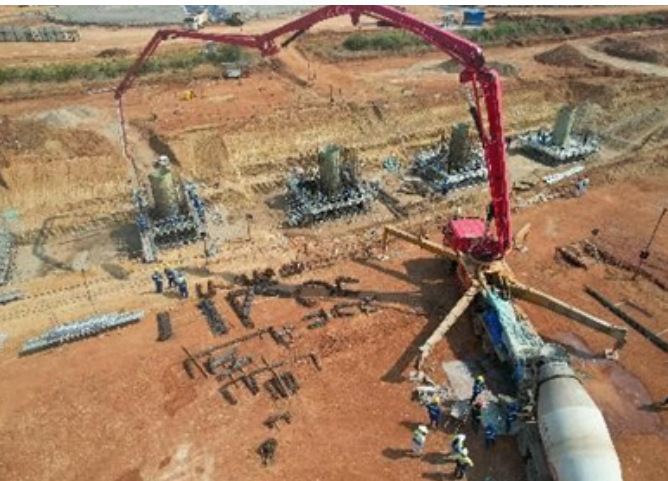
Marine Terminal Recirculation Pump concrete casting
