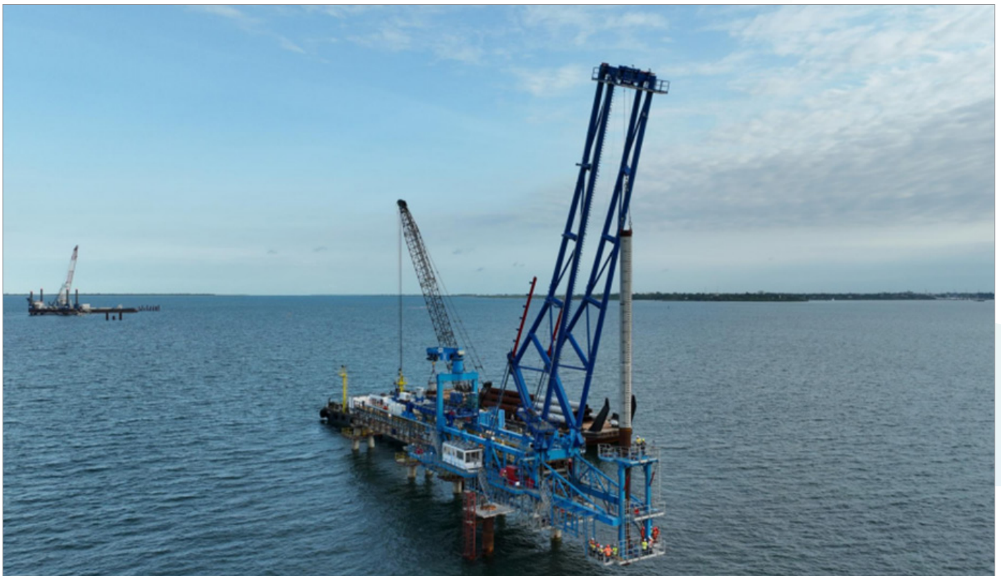
Jetty Launching Girder 1st pile installation
