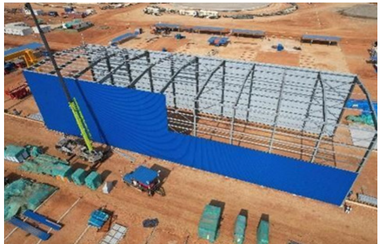
Marine Terminal Construction Workshop installation
