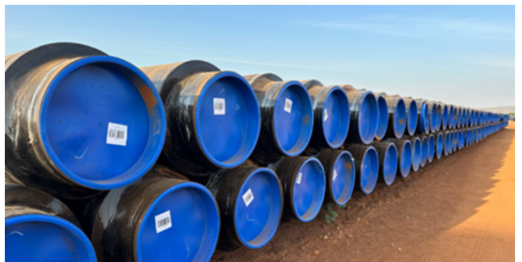
PUF pipe stacking
