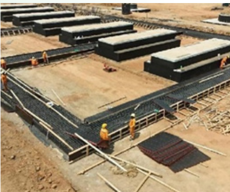
PS-4 Power Gen building rebar fixing
