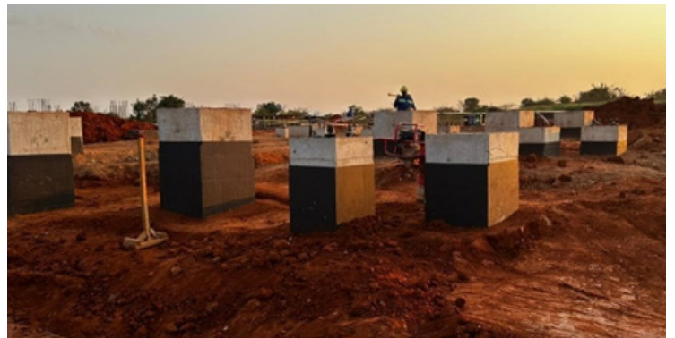
PRS-2 Pipe Support backfilling
