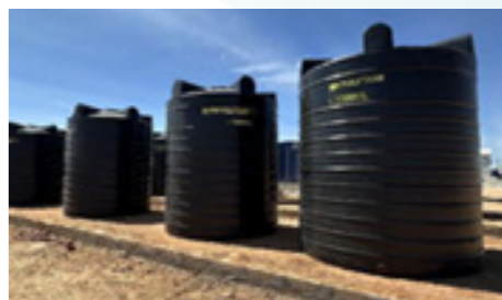
5 water tanks arrived and were unloaded
