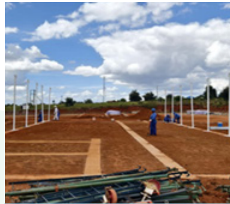
Traning Center Posts erection
