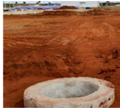
Sewage Network Backfiling
