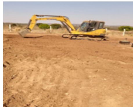
Backfilling work in progress around Septic tank
