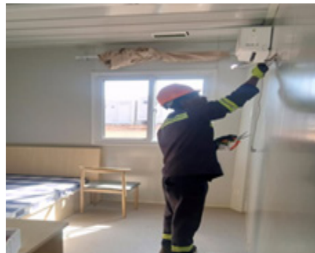
AC, Furniture and Electrical work in progress for Of Bed Room
