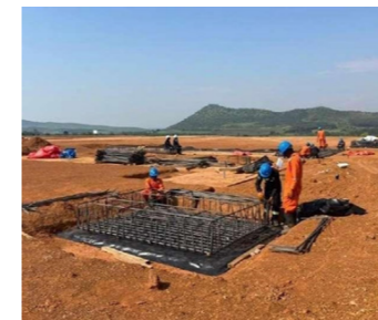
PS-1 Metering Package rebar fixing
