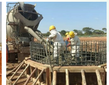
PS-4 Exhaust Stack concrete casting
