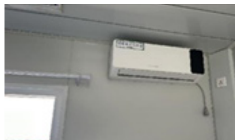
Air conditioning installation in double room dormitory
