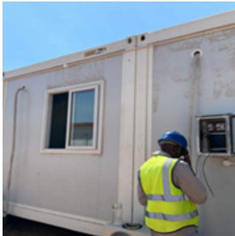
Single/Double and Four Bedrooms Cable Testing for Wifi Router
