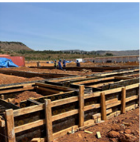
Training Center Type 1 Formwork Fixing
