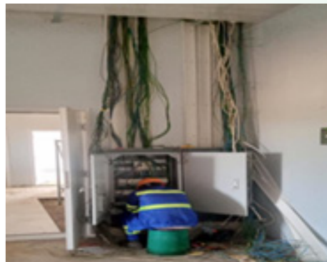
Electrical work in progress for canteen type 1
