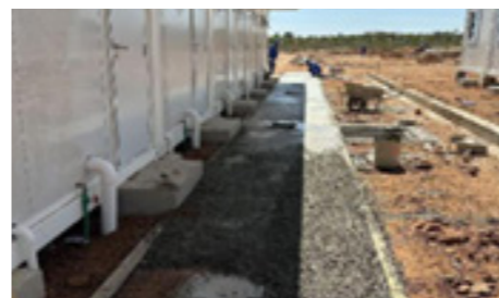
Construction of sidewalks en single and double dormitory areas
