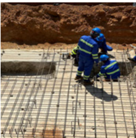
Shaft Tank Foundation Steel Fixing
