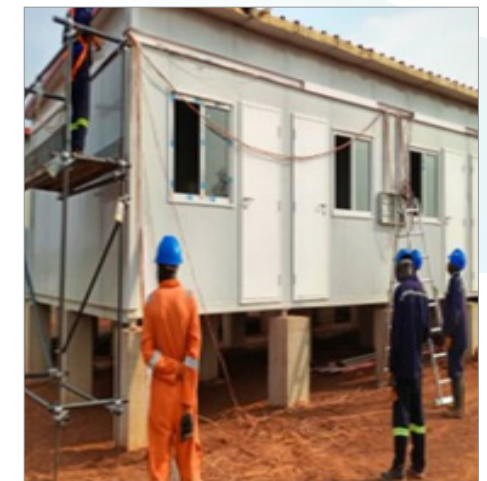
Installation of supply cables for AC Circuits and lighting ccts.
