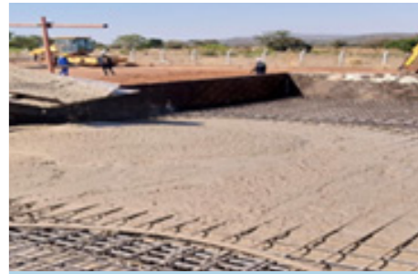
Concrete work in Progress for Sewage Holding tank (Top slab)
