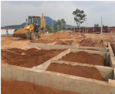
Backfilling for CTR office type 4
