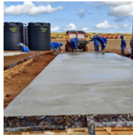
Water Tara Top binding of platform
