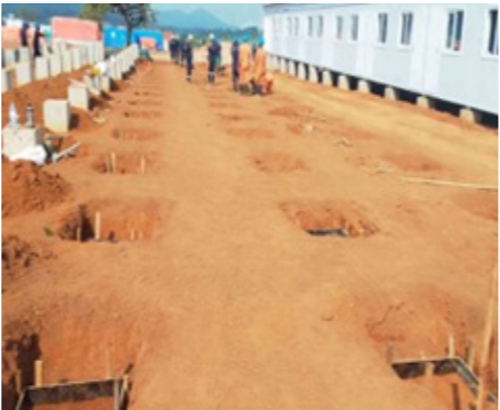
Fixing formwork for blinding concrete for four bedroom dormitory block 3
