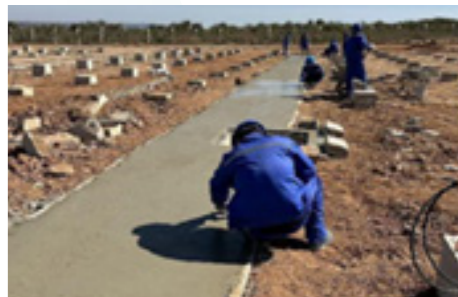
Construction of sidewalks in the four-person dormitory area
