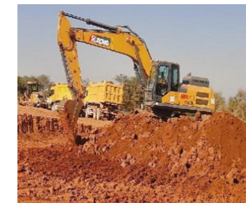
PS-3 Cut works
