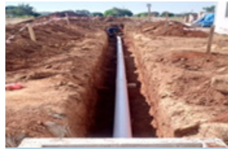
Pipe line installation work in progress for sewage water
