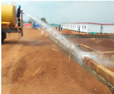
Concrete curing for CTR canteen 2 type 1
