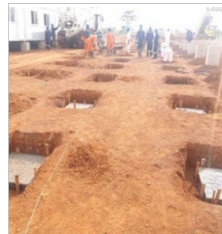
Casting blinding concrete for fourbedroom dormitory block 3.
