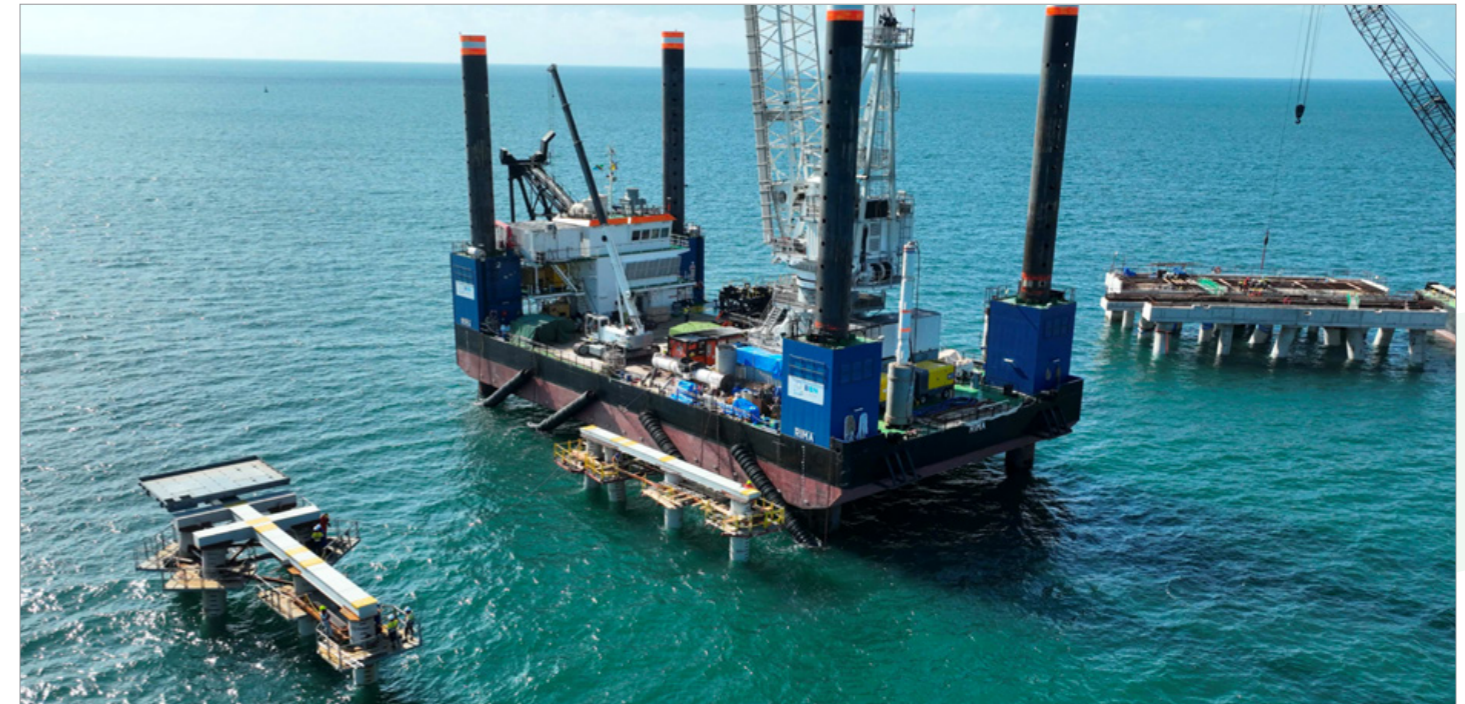
Jetty Crosshead installed at EITS platform
