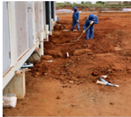
Sewage Network Backdilling
