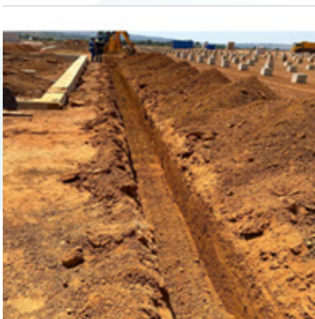
Excavation for Earthing and Power Cables
