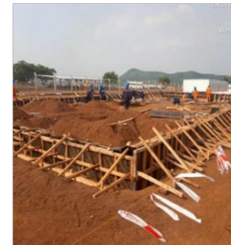
Shuttering and fixing formwork for CPY office type 2.
