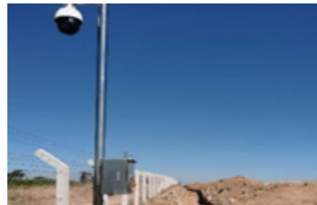
Install CCTV equipment
