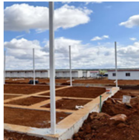
Training Center Posts erection
