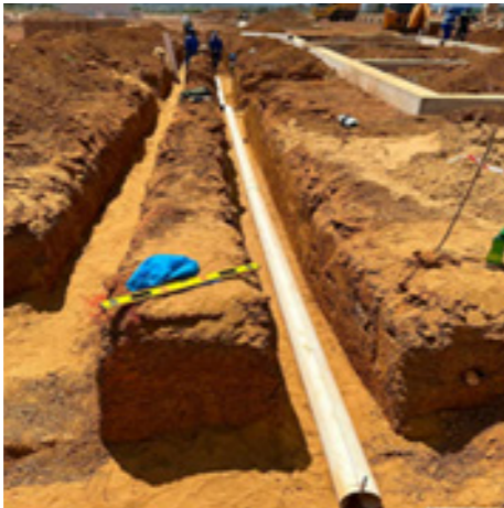
Sewage and Water Supply Laying of Piping and Sand Filling
