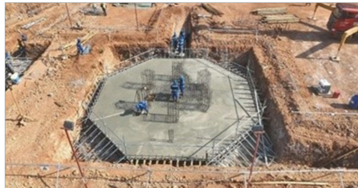
Marine Terminal Direct Fired Heater foundation concrete casting
