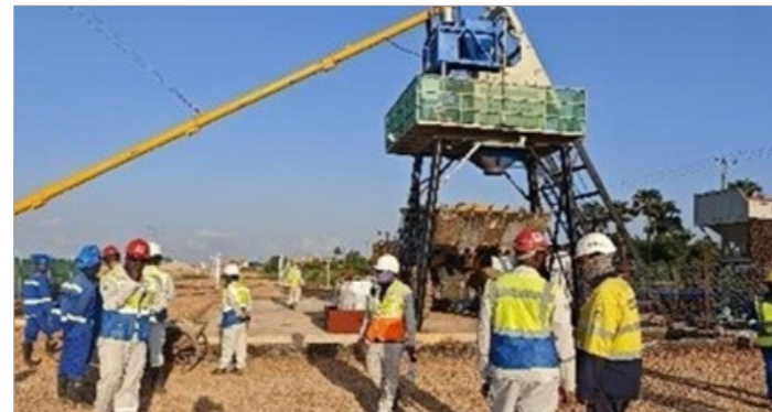
Marine Terminal Batching Plant commissioning
