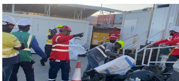
BBN workers cleaning Marine base (laydown area).
