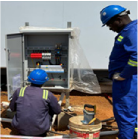
Fixing of Electrical Distribution Box MCPY06 - DB05, 04, 03, 02, 01
