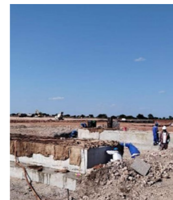
PS-5 Export Pump foundation curing
