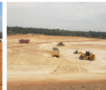
PS-2 cut works
