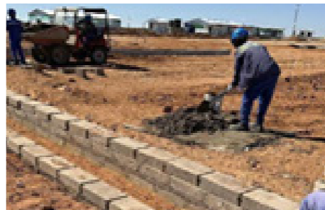
Construction of drainage ditch in the insemary area
