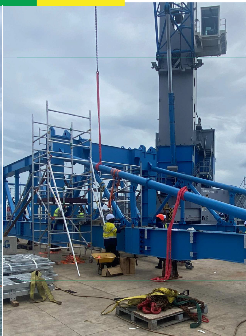
Ongoing Launching Girder Assembly
