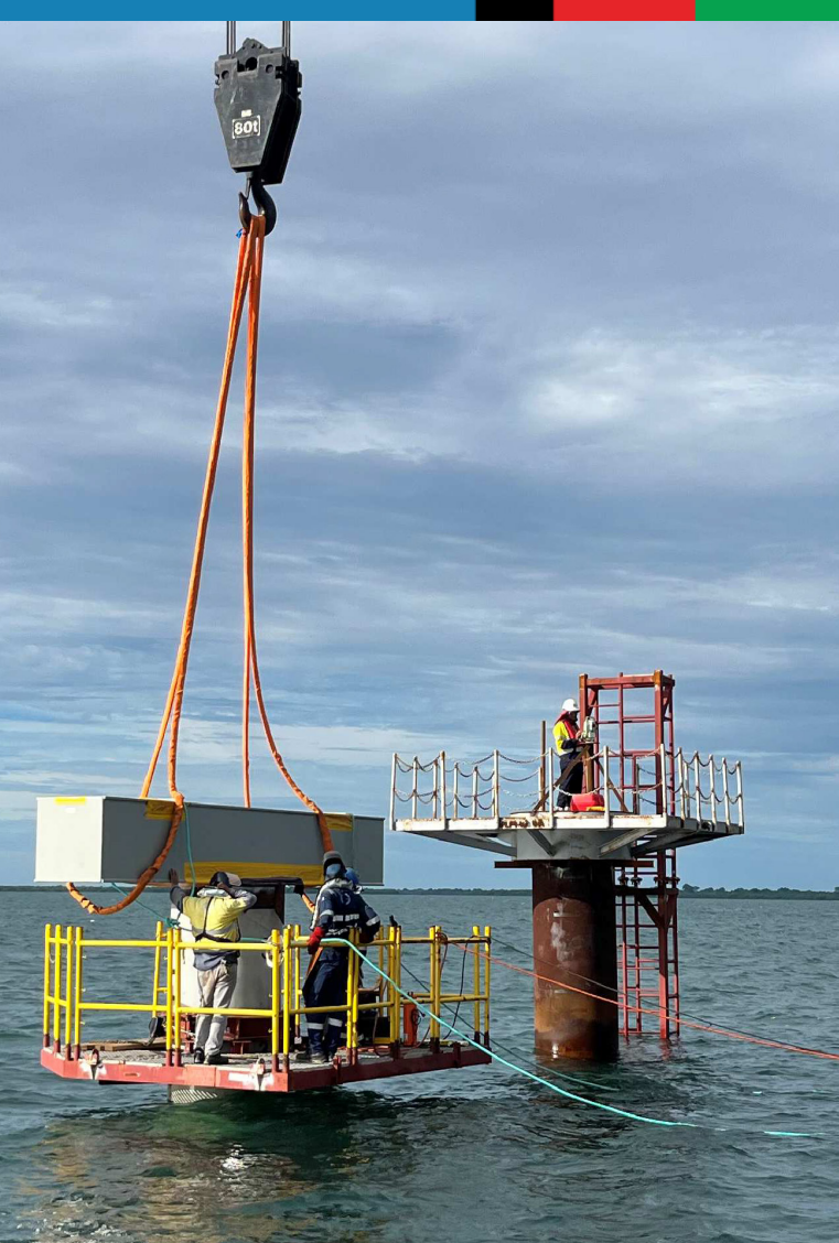
First Crosshead Installation
