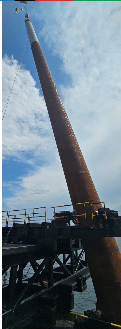
First 2 raked piles of the Loading Platform of the Jetty
