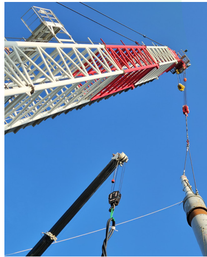
First 2 raked piles of the Loading Platform of the Jetty
