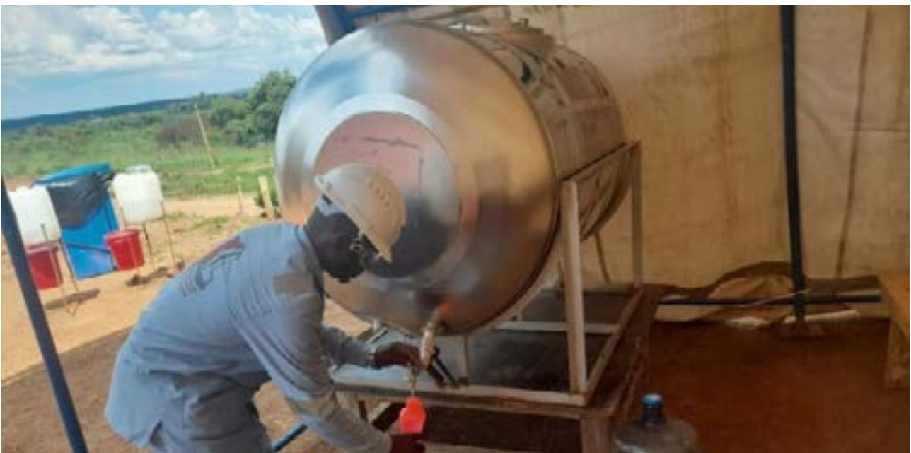
Figure 12: Portable drinking water at site
