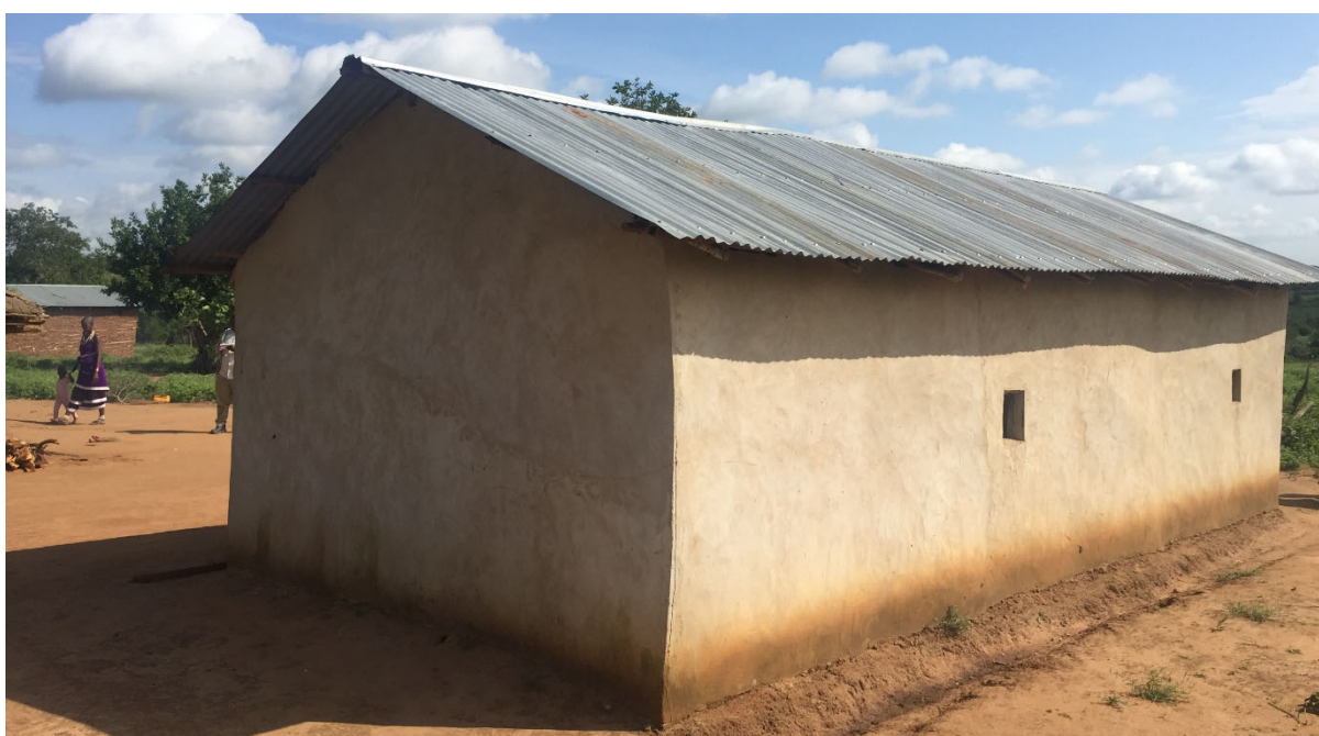
Figure 7-3: Modern House of Plaster Block and CIS roof in Kilindi
