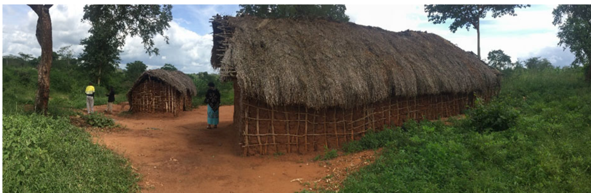
Figure 7-1: Traditional House in Handeni Constructed from Mud and Poles with a Thatch Roof
