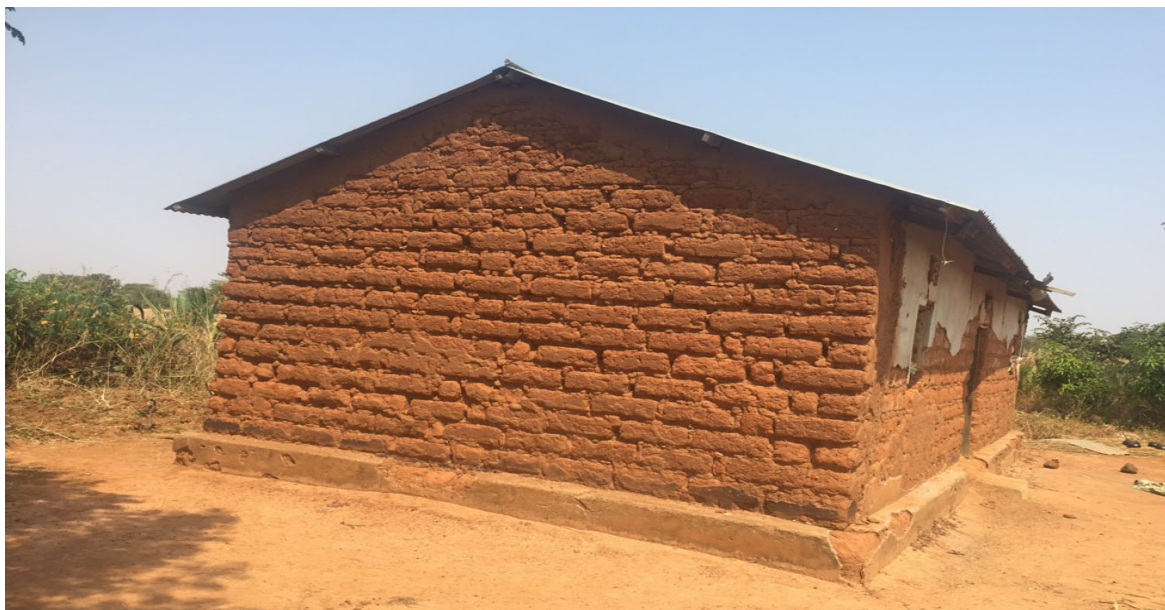
Figure 7-3: Traditional Mud Brick House with Modern Roof in Nzega
