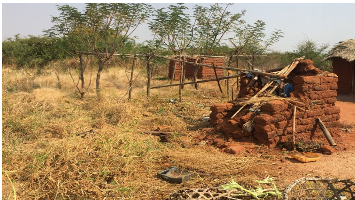
Figure 7-6: Example of a Toilet Structure Found in Nzega
