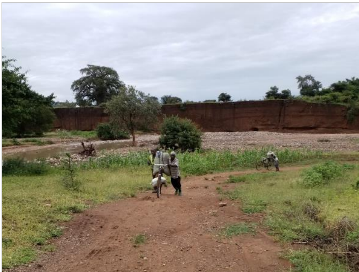
Figure 5-21: Example of poor road infrastructure in Mtoa Ward
