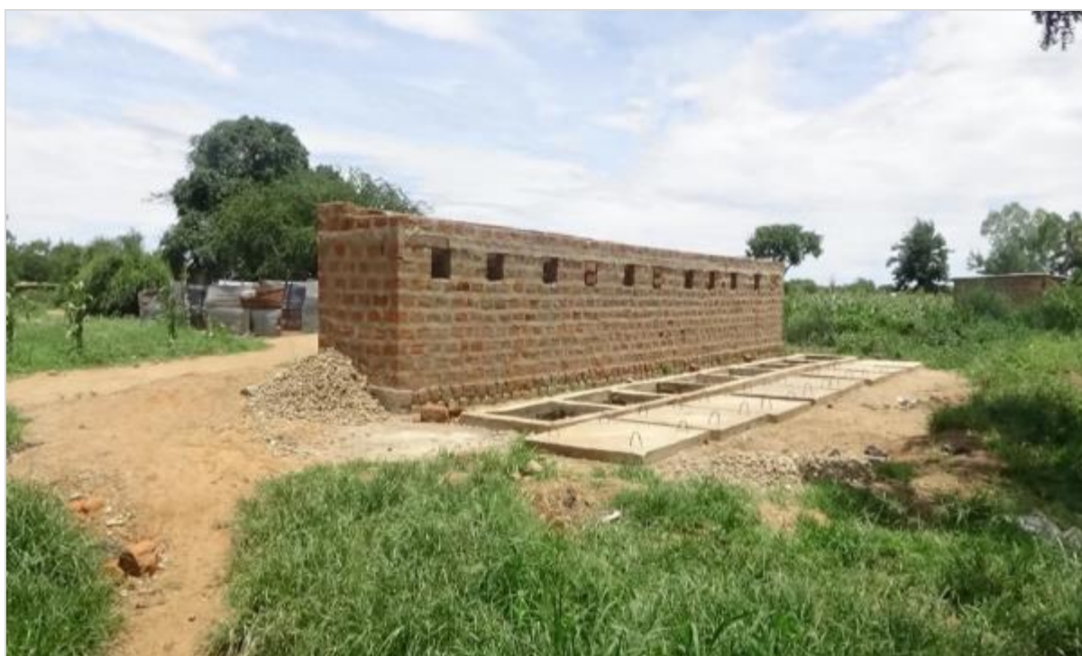
Figure 5-18: Construction of improved pit latrines underway in Mtoa Ward (Iramba District)
