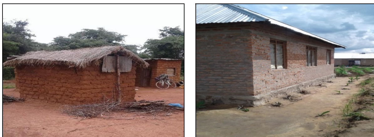
Figure 7-1: Examples from Shinyanga Region of a typical traditional mud, brick and thatch tembe house (left) and a modern house of burnt brick and CIS roof (right )
