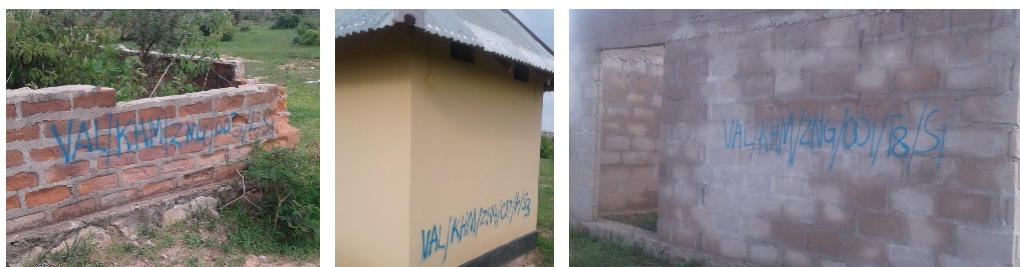
Figure 4-4: Examples of Valuation numbers placed on dwellings and structures as part of the survey process.
