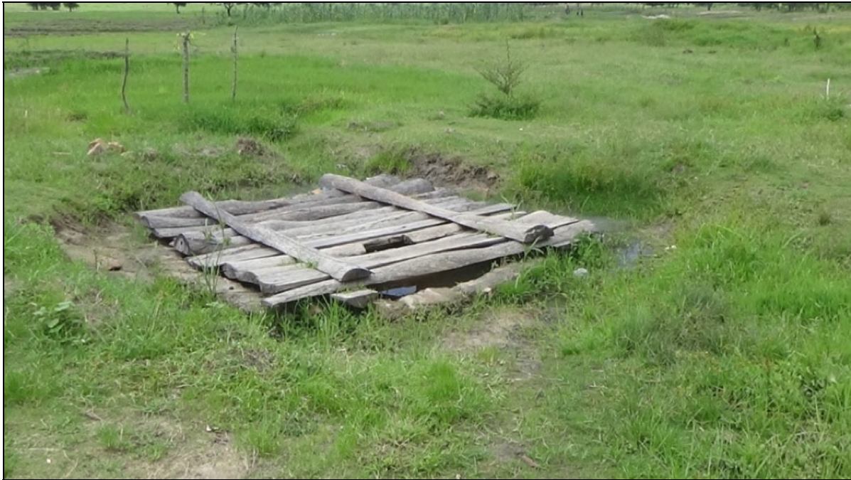
Figure 5-9: Example of a Covered (Protected) Communal Water Well (Wendele Village)
