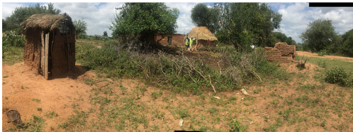
Figure 7-8: Example of a Toilet Structure Found in Manyara Region
