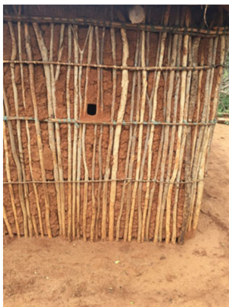
Figure 7-5: Small Opening in a Maasai House in Kiteto, Providing Limited Light and Ventilation
