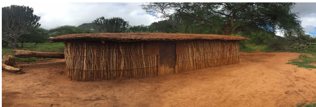
Figure 7-4: Example of a Traditional Maasai Oval Shaped Residential structure in Kiteto
