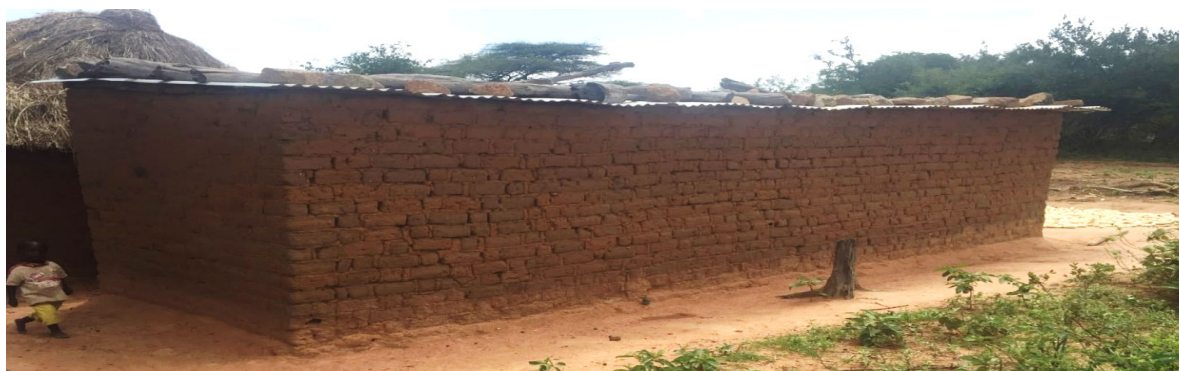
Figure 7-3: Traditional Mud Brick House with Modern Roof in Hanang
