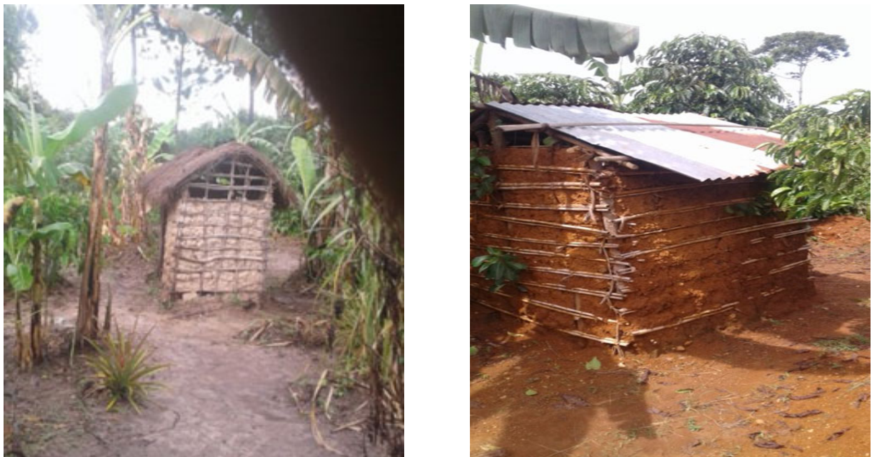
Figure 7-5: Examples of toilet structures found in Kagera Region
