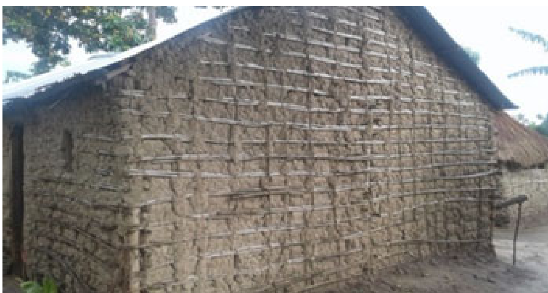
Figure 7-2: Example of traditional mud brick house with modern roof
