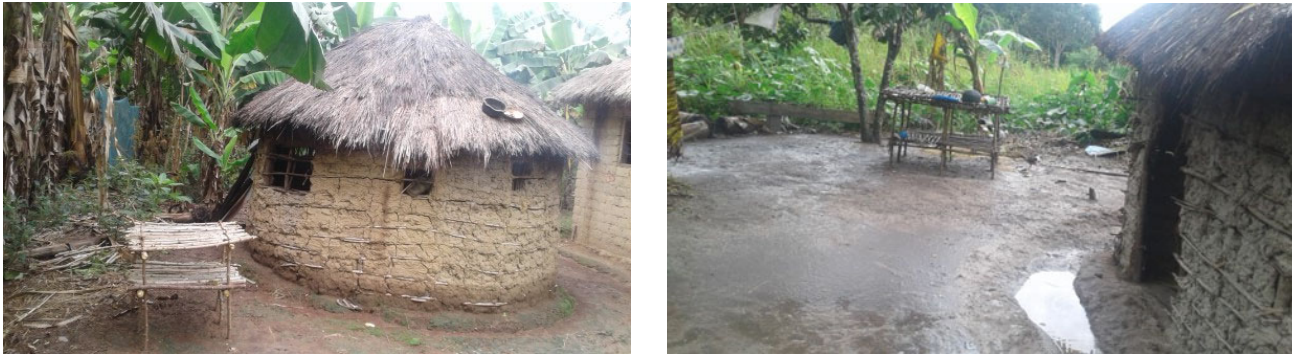
Figure 7-4: Examples of kitchens found in Kagera Region
