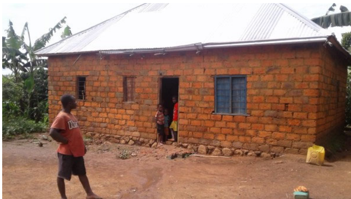
Figure 7-3: Modern house in Kagera with stone foundation, burnt brick and CIS roof
