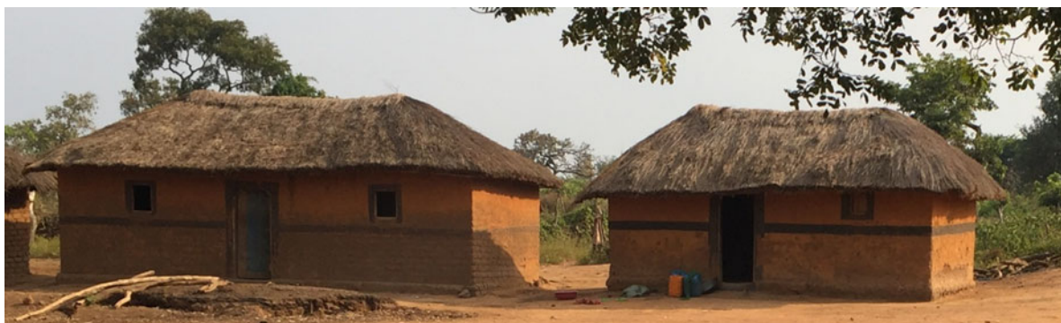
Figure 7-1: Traditional House Constructed from Mud Brick, Mud Mortar and Thatch Roof in Geita District
