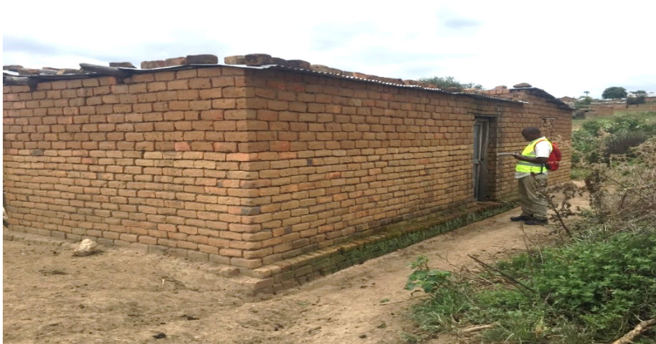
Figure 7-3: Example of Burnt Brick House with a Modern Roof from Kondoa
