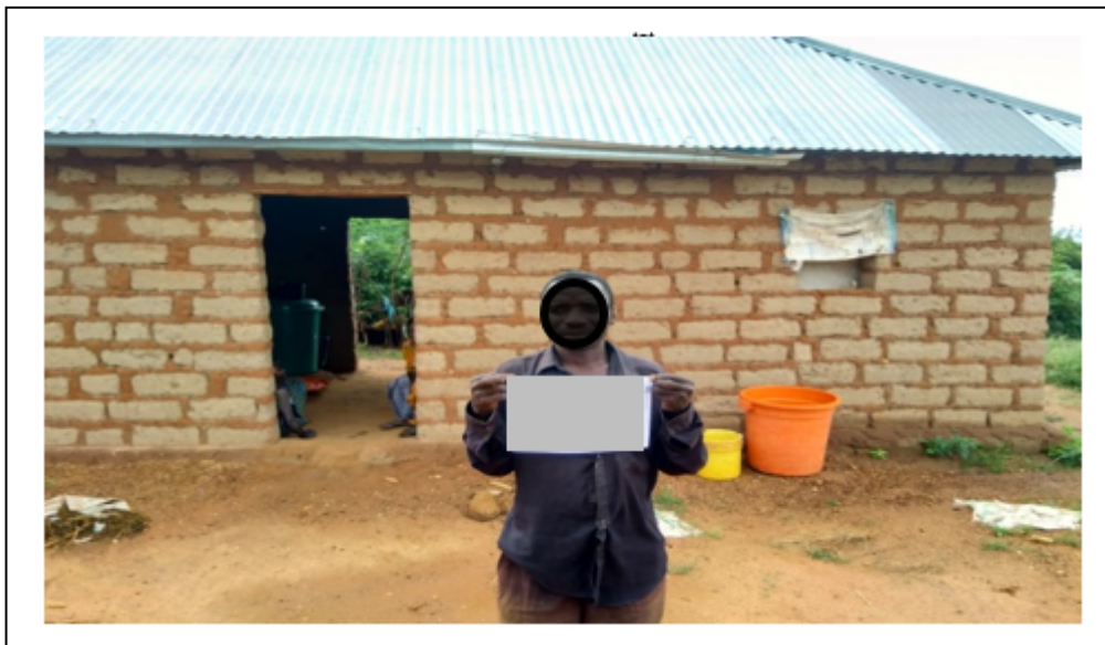
Figure 6-3: Example of a modern house (burnt brick and corrugated iron sheeting)
