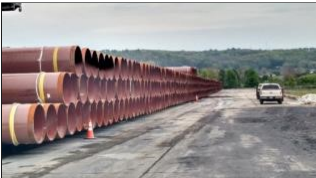
Figure 2-21: Example of a Typical Pipe Storage Yard
