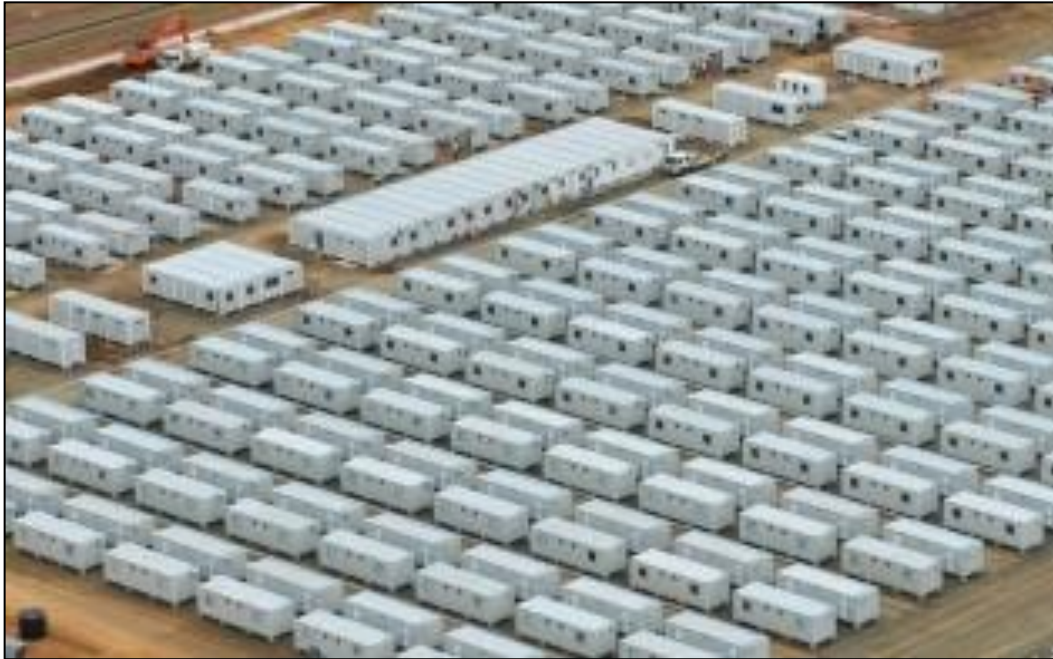
Figure 2-20: Example of a Typical Construction Camp with (Temporary Office and Accommodation Facilities)
