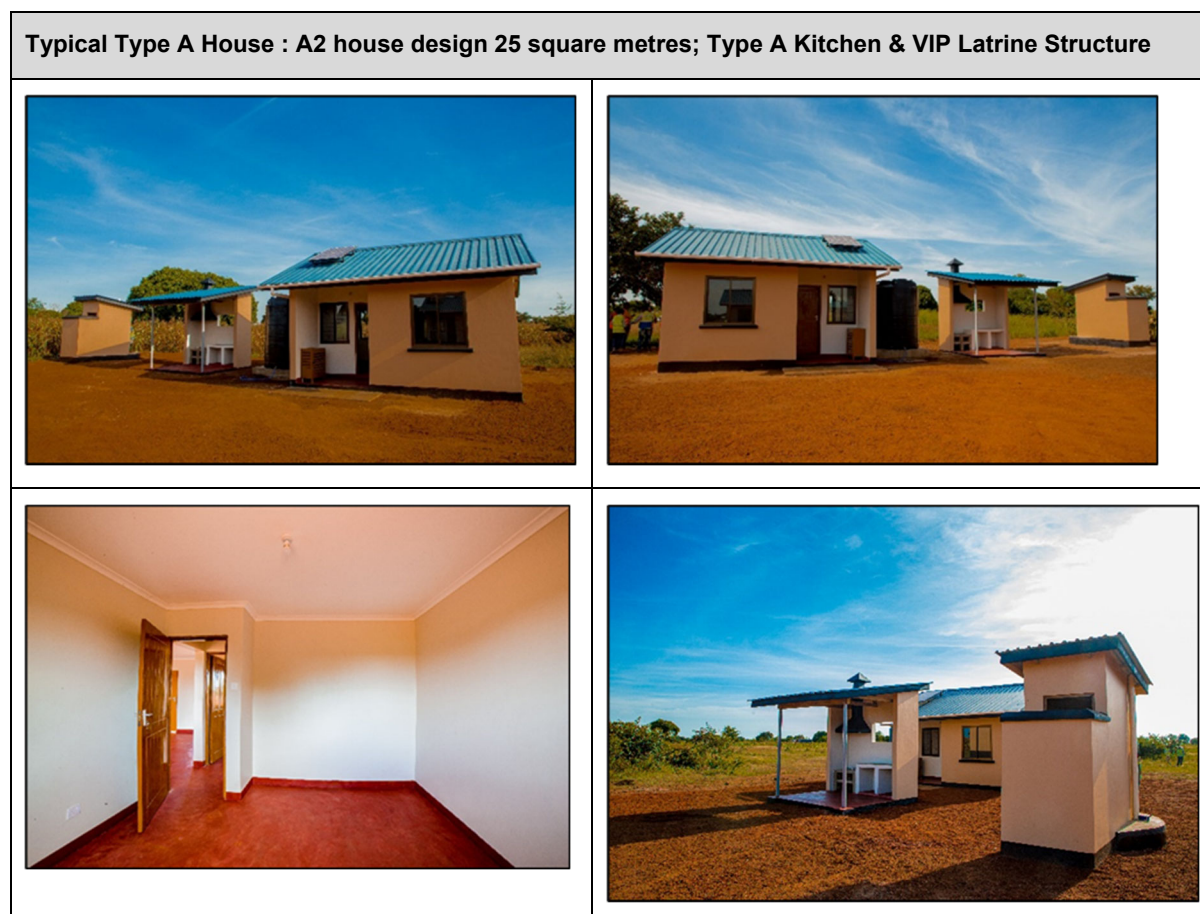
Figure 6-1 Example Completed Replacement Housing (Type A)
