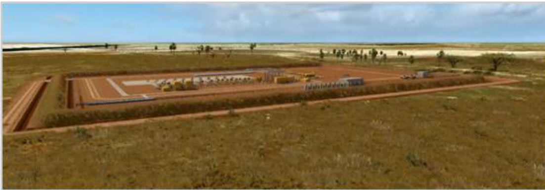
Figure 4: Visualisation of a well pad in the MFNP with outer ditch and screening bund wall (Source EACOP MFNP Well pad Visualisation Projet_U_V0.5)
