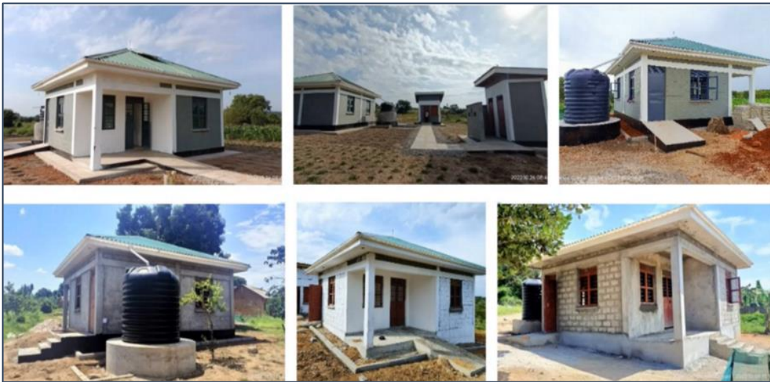
Figure 12: Examples of replacement housing nearing completion in Uganda (Source: EACOP, 2022)
